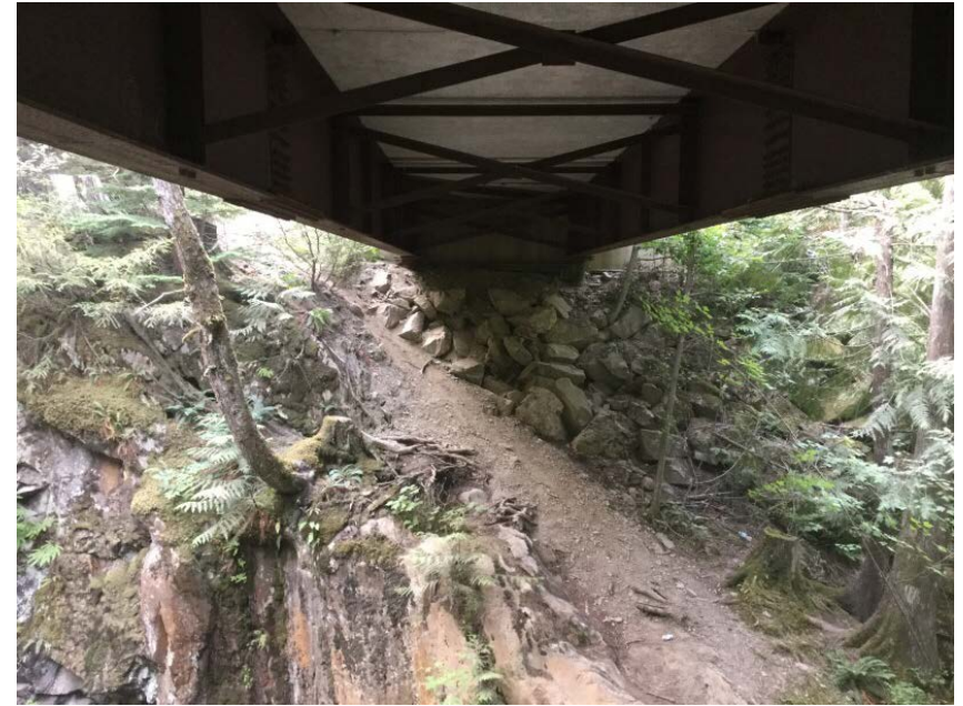
Left Bank Abutment when facing downstream
