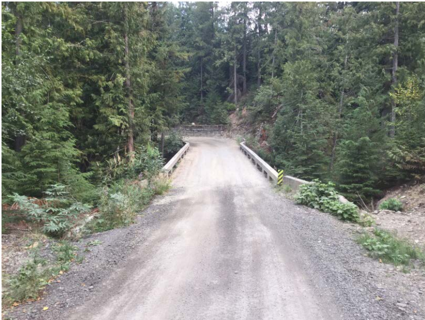
Approach from Left Bank when facing downstream
