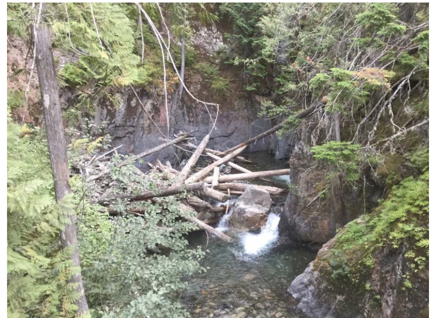
Looking upstream from deck
