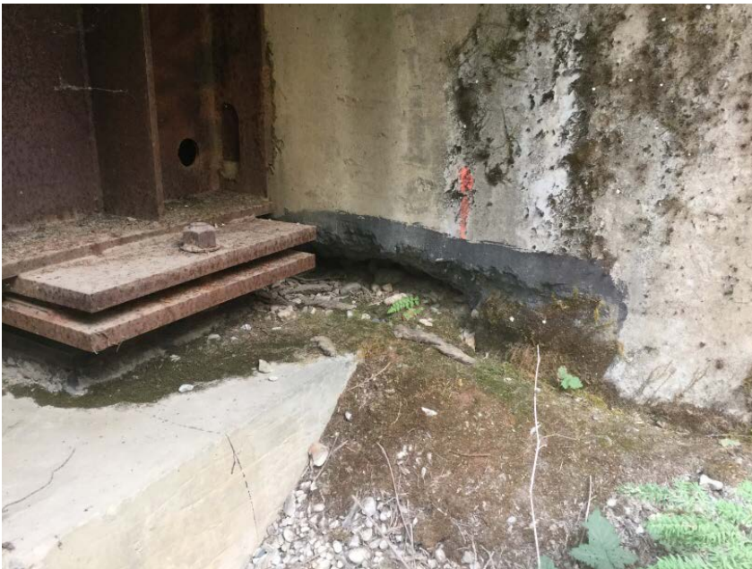
Ballast Wall at upstream right bank
