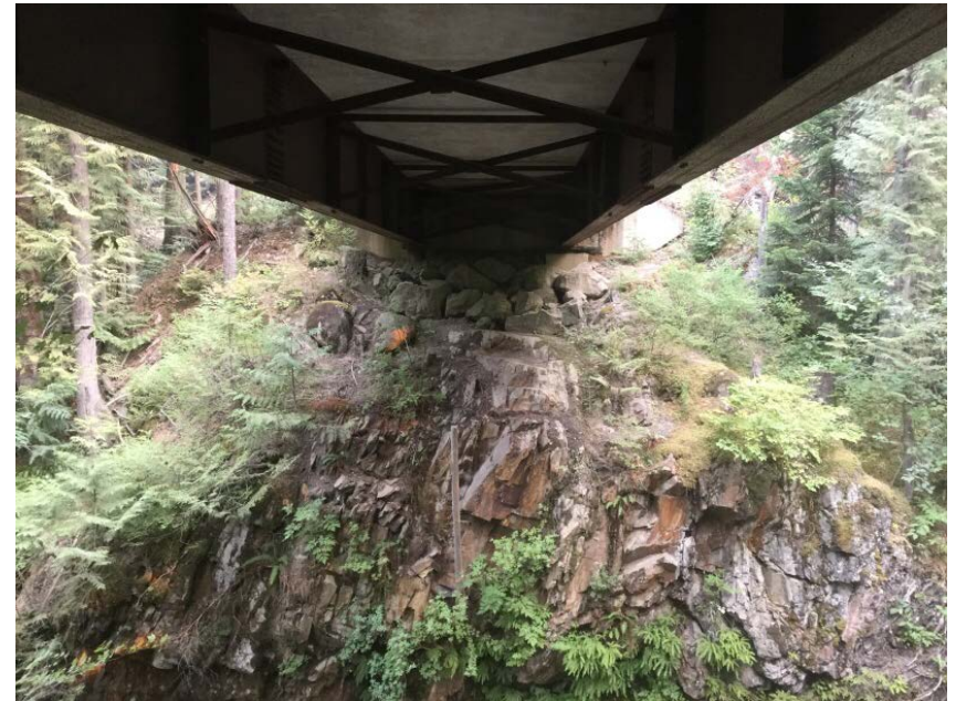
Right Bank Abutment when facing downstream
