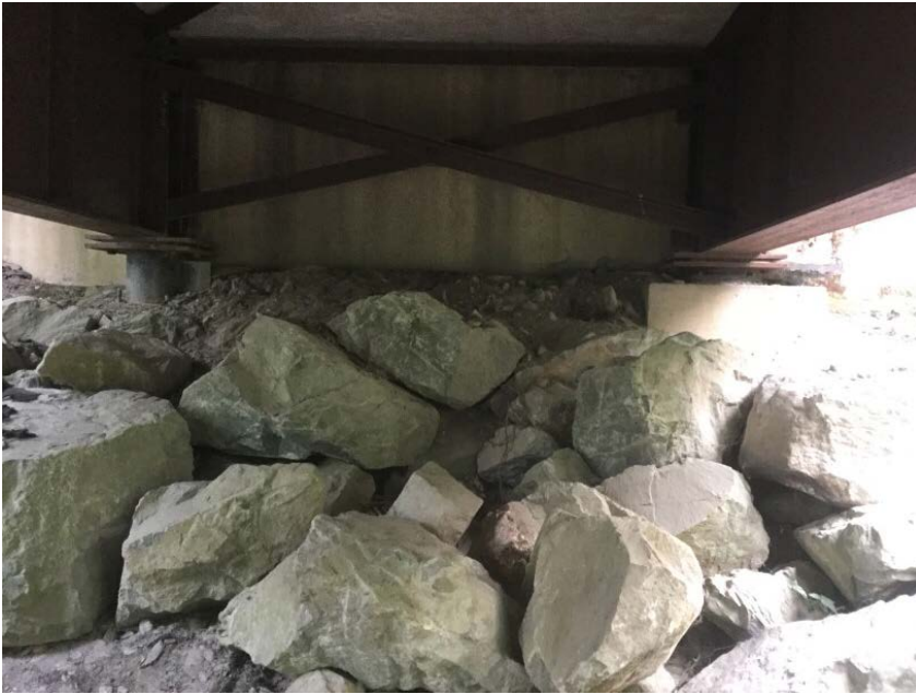
Right Bank Abutment when facing downstream
